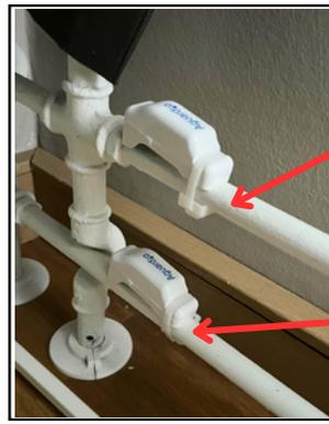
A. PLACE THE PIPE SENSOR ON THE INLET PIPE TO THE RADIATOR
