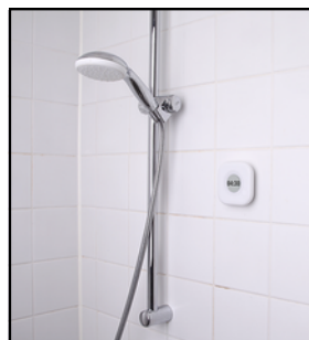
Positioning of the Shower Sensor
